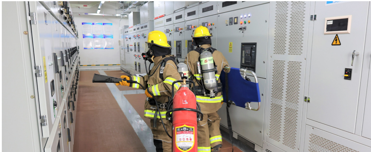
In April 2022, the Company organized an electrical fire emergency drill
