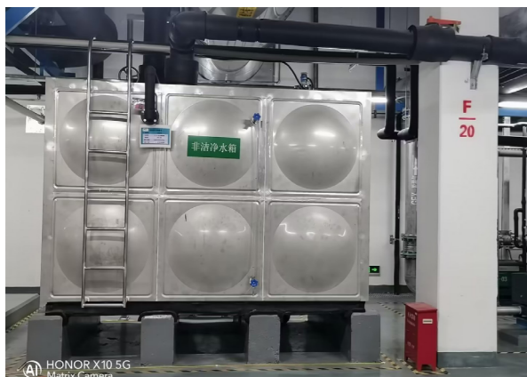
The introduction of condensate recovery system can collect condensate from the plant air conditioners for reutilization, effectively reducing water consumption.
